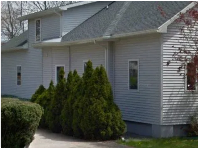
My perch, 40-some years ago, after some significant renovation, and shrubs.
